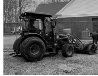
Sidewalk repairs at Town Hall
