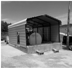
New fuel pump shelter
