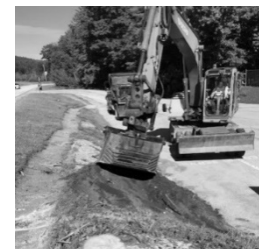
Swale at Safety Complex
