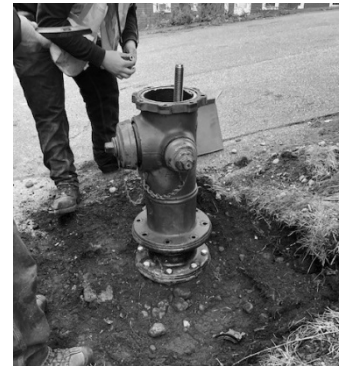
Replacing hydrant on Abbey Rd
