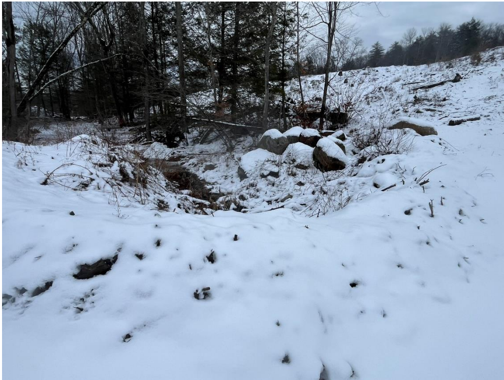
Rip-rap and filter berm maintained at wetland crossing culvert
