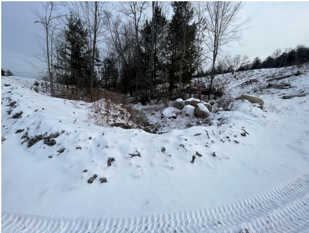
Frozen wetland protected by filter berm
