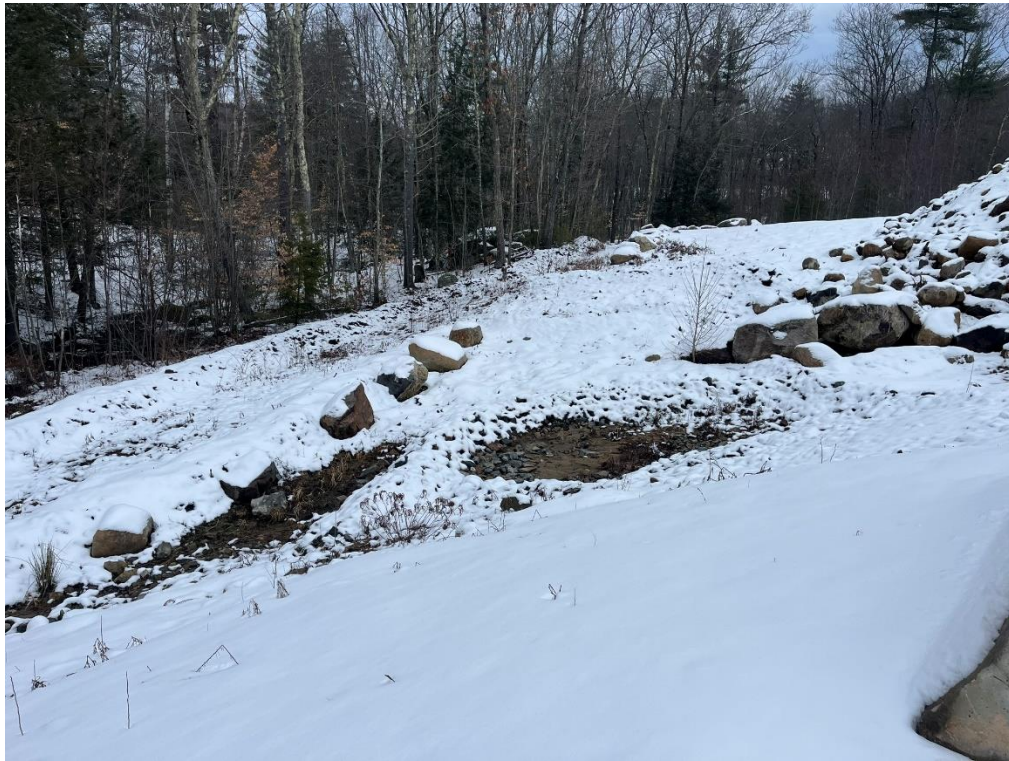
Filter berms maintained
