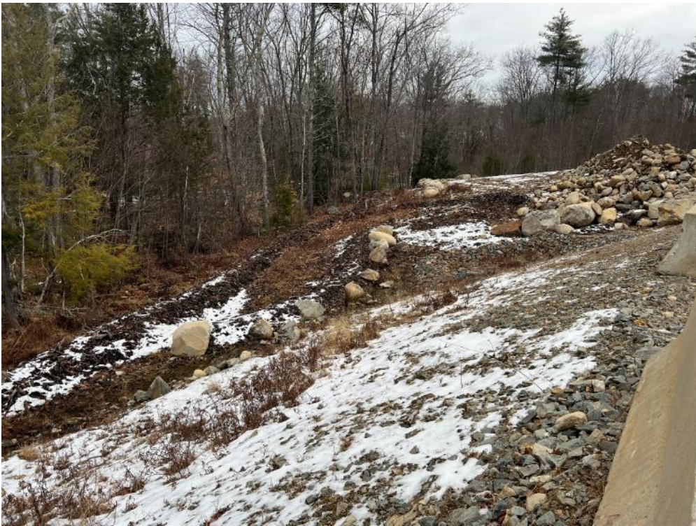
Double filter berm at low point
