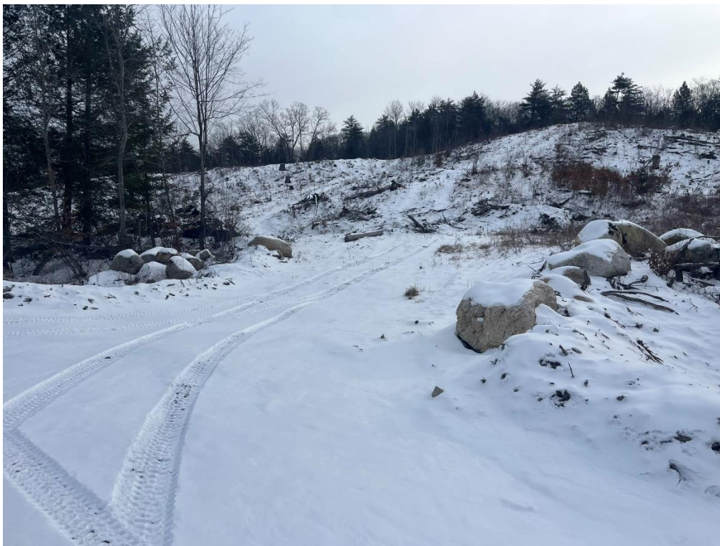
Wetland crossing – filter berms maintained
