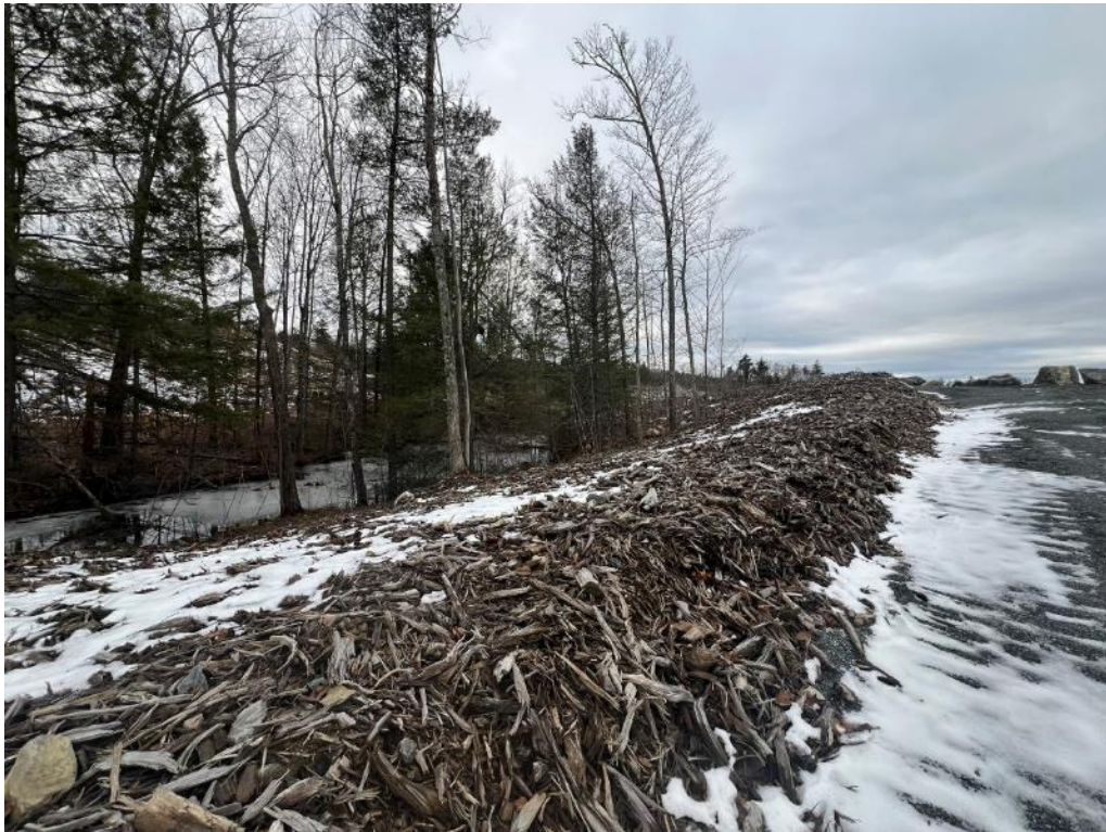
Stabilized slope at wetland pocket
