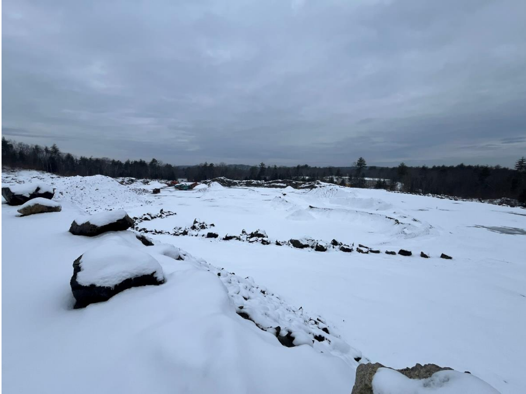
Typical site conditions in gravel pit
