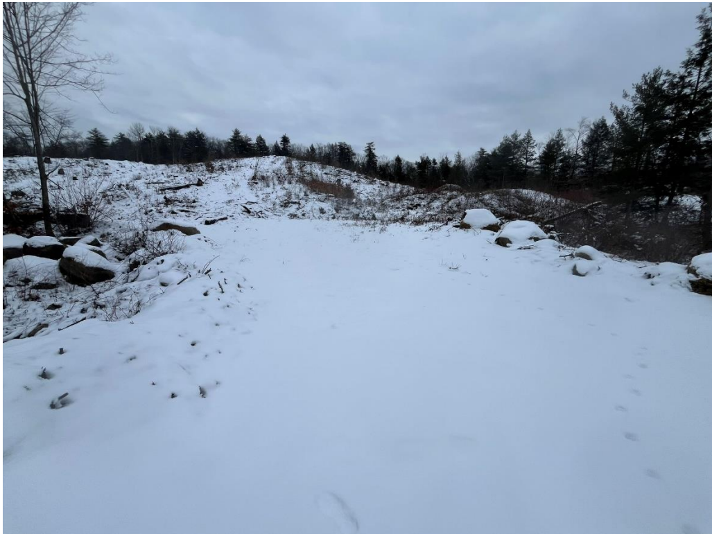
Wetland crossing – filter berms maintained
