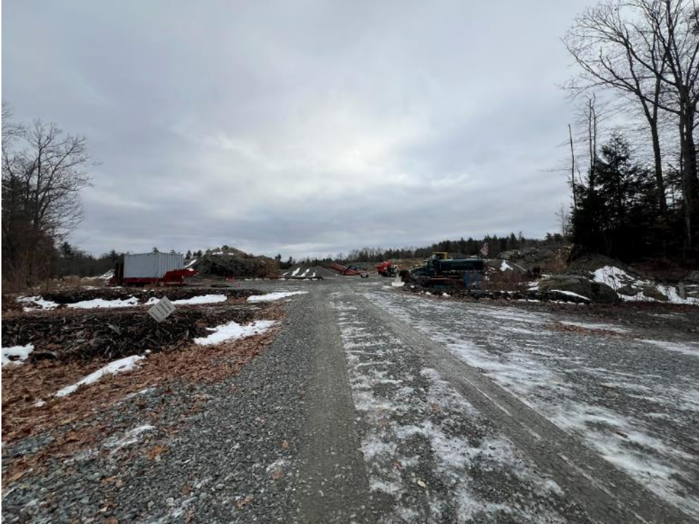
Check dams at site entrance
