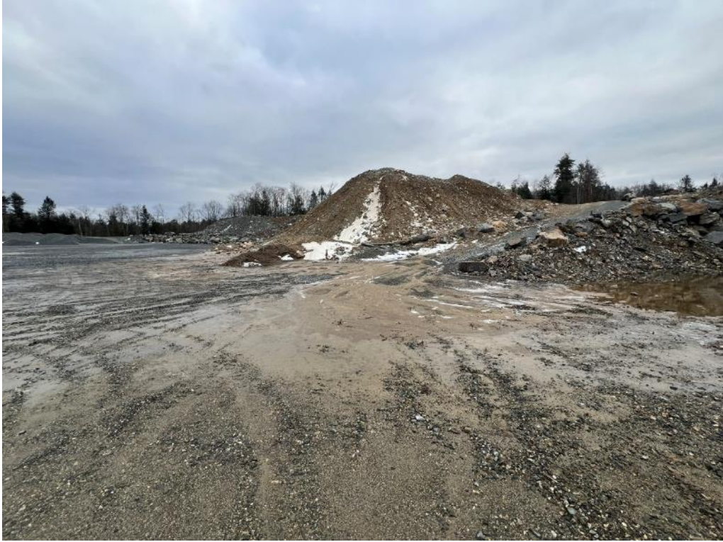
Silt contained to base of stockpile
