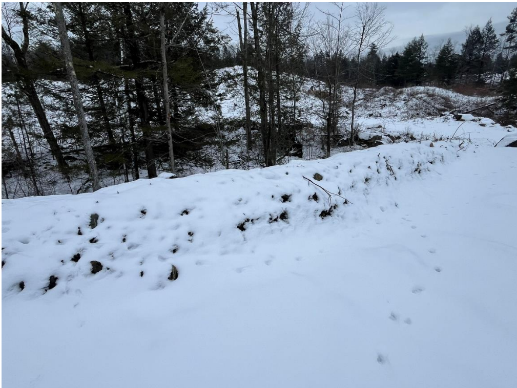
Frozen wetland protected by filter berm
