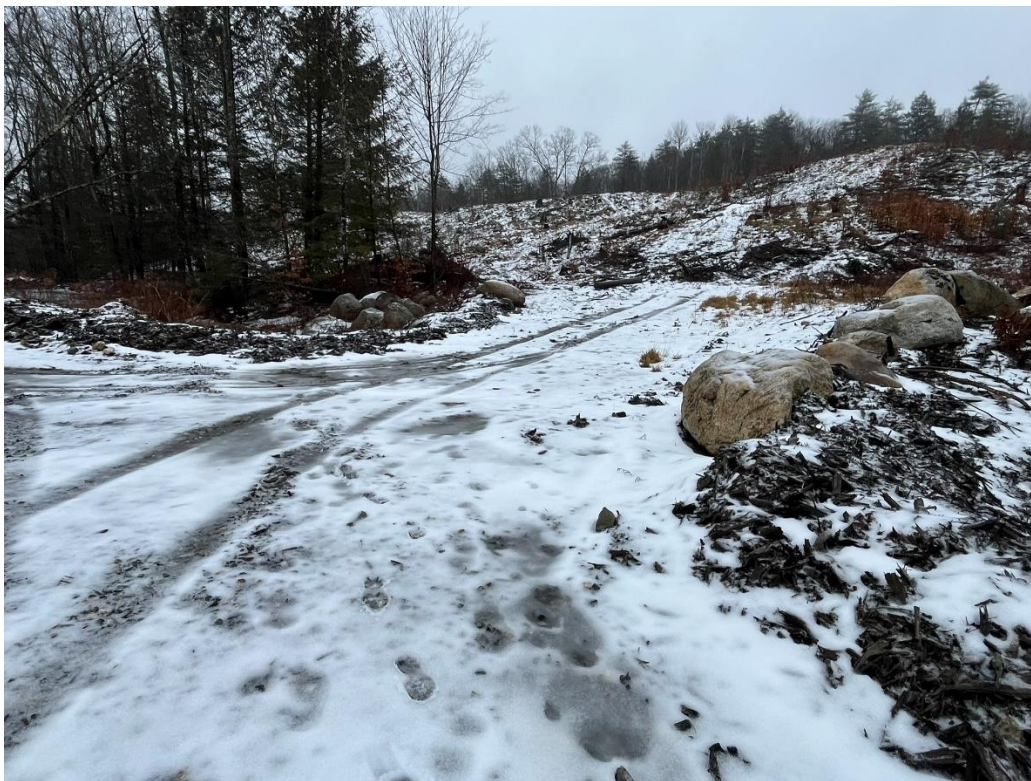
Wetland crossing – filter berms maintained
