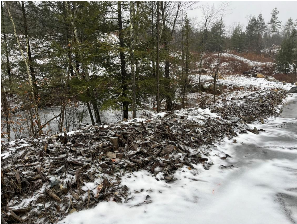
Frozen wetland protected by filter berm
