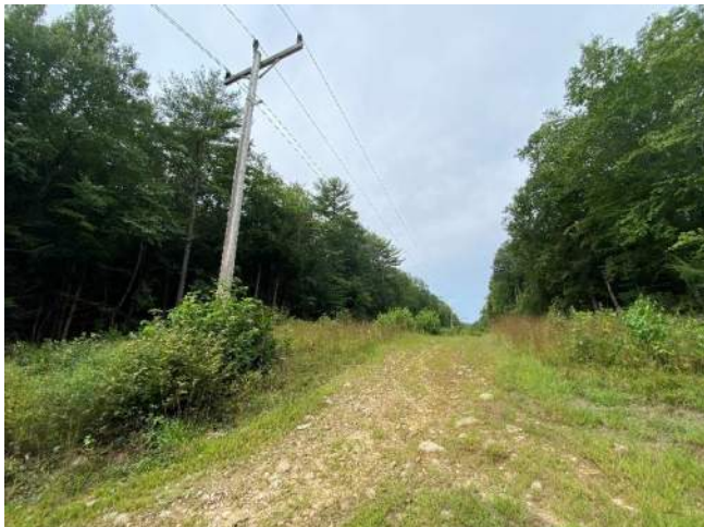
Description: Electrical line running through Target Property.
