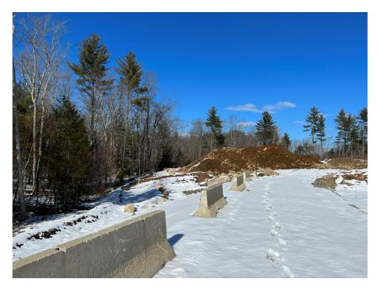
Plunge pool and double filter berm at edge of disturbance
