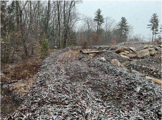
Plunge pool and double filter berm at edge of disturbance
