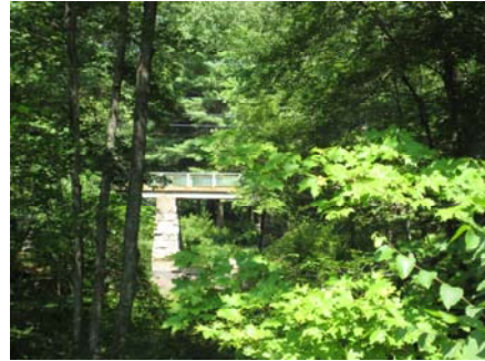
Dudley Road Stone Bridge
