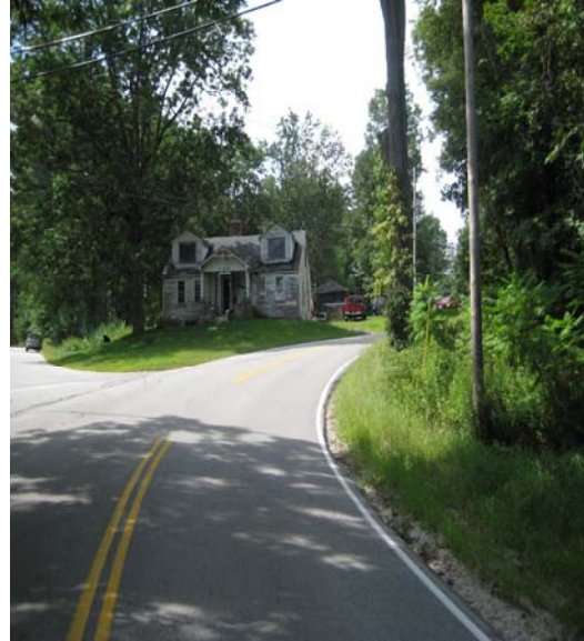
Limited Sight Distance- Lane Road at Shattagee Road
