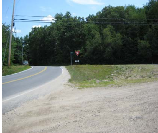
Eastbound Scribner Road Approach to Gile Road- Confusing Signage and Evidence of Use of Shoulder for Turns
