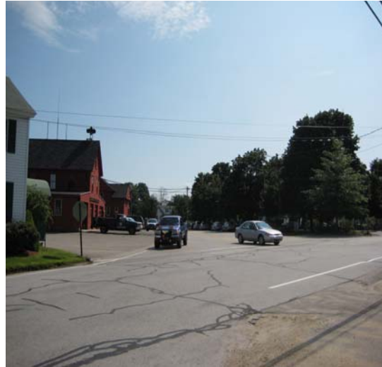
Excessive Pavement Width- Epping Street Approach to Main Street
